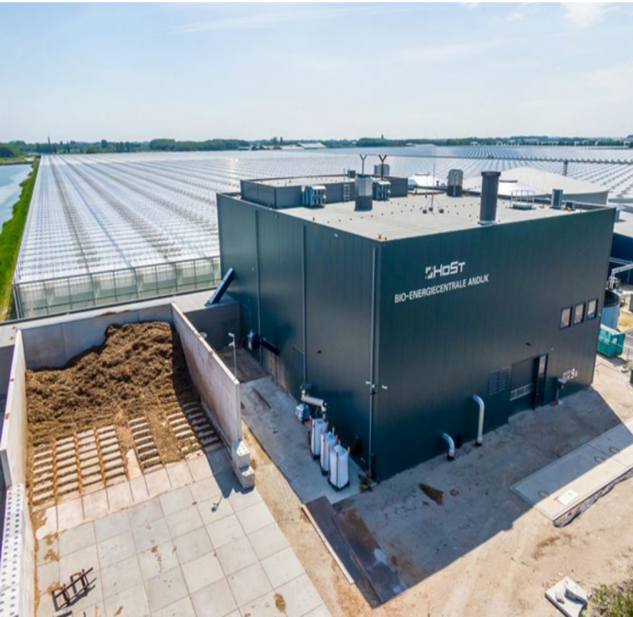
HoSt's 2020 State-of-Art Biomass CHP Plant: Produces 15 MW thermal + 3.4 MW electrical power
